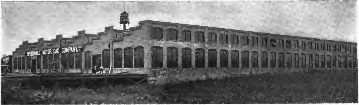
Addition to Plant of the Speedwell Motor Car Company, Dayton, O., That Will Be Followed by Another of Similar Size
